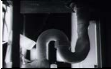
Shot 15 cont. The camera descends and shows some object making a bulge in the drain pipe as it passes through.
